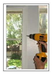
Attach the shutter panel to the frame using the hinge pin to hold them in place. The shutter panel with the "Lip" should be installed on the right side of the frame.
