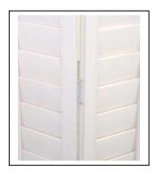
7. Any minor gaps at the corners & predrilled screw holes should be filled with caulk and color matching touch up paint. (included)
